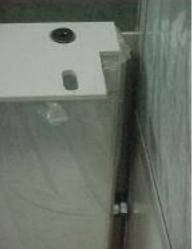
34) After fitting the gable end assembly in the panel, adjust the hex head screw with the help of flat spanner such that the screw head touches to the panel.
