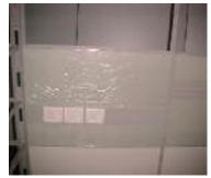
18) Slide in the accessory rail in to the panel no. 4 & 5 as per the following sequence of tiles - 315mm ht. tile, accessory rail & 150mm ht. tile
