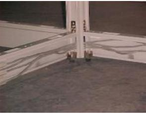
12) Fit vertical trim of 1200 mm Ht. to the panel no.4,5 & 6 with the help of M6 x 20 mm fixed screws
