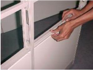
16) Slide in the tiles to the 2<sup>nd</sup> module. Ensure that tile supporter catch fitted to tile is perfectly engaged with the tile supporter on pipes
