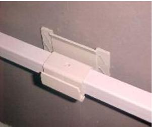
17)Fit the power beam in the  $2^{\rm nd}$  module & follow the following sequence of the tiles - 150mm Ht. tile, power beam & 315mm ht. tile
