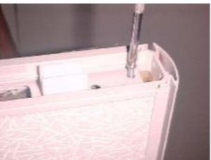
20)Take out the glass tile accessories i.e horizontal & vertical cover (2 nos. of each) which are to be fitted in 3<sup>rd</sup> module of 1500 height frames.
