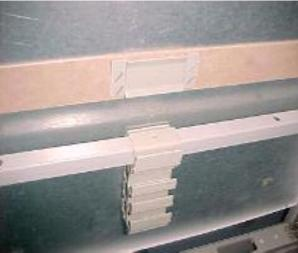
15) After fitting all the lower tiles in first module, put on the tile holders wherever required
